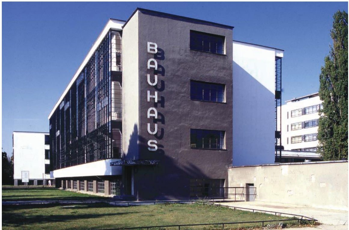
FIGURE 3.17 The Bauhaus School of Design (1925–26) is a prime example of the emerging Modernist style at that time. The building design is functional, utilitarian, and devoid of ornamentation.
