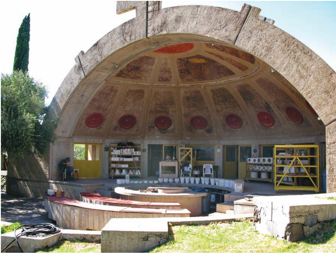
FIGURE 10.3 Associates of Paolo Soleri are constructing one of his visionary cities, "Arcosanti," in Arizona. CC-BY-NC-2.0/Alan English
