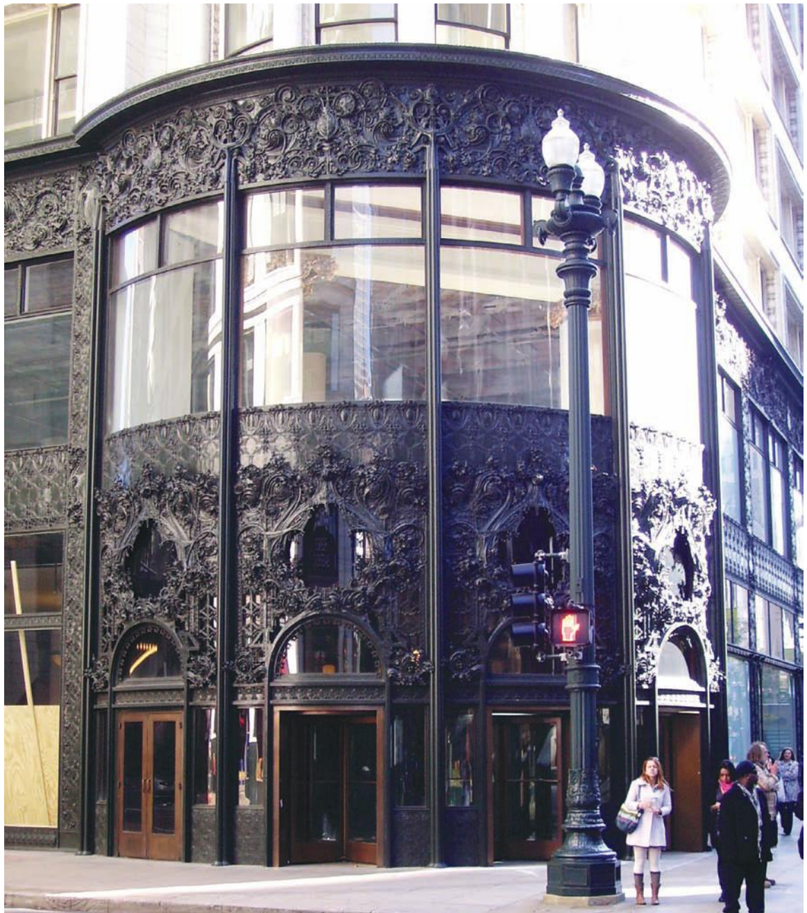
FIGURE 3.10 Louis Sullivan designed the tracery around the street-level windows of the Carson, Pirie, Scott and Company Store (now the Sullivan Center) in Chicago (1901–1904). His designs reflected the art nouveau influence of nature-based motifs. Look closely and you will find his initials in the design.
