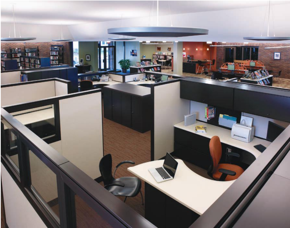
FIGURE 12.35 Successful office lighting incorporates more than one type of system for interest and visual relief, including indirect lighting to reduce direct glare.
