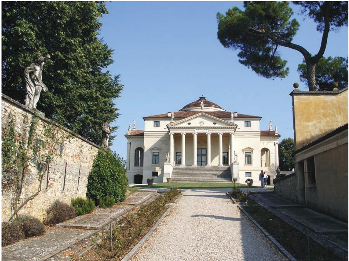
FIGURE 2.24 Andrea Palladio's Villa Rotonda (1550) on a hill near Vicenza, Italy, has a central domed salon that is symmetrically flanked on four sides by identical projecting porticoes.
