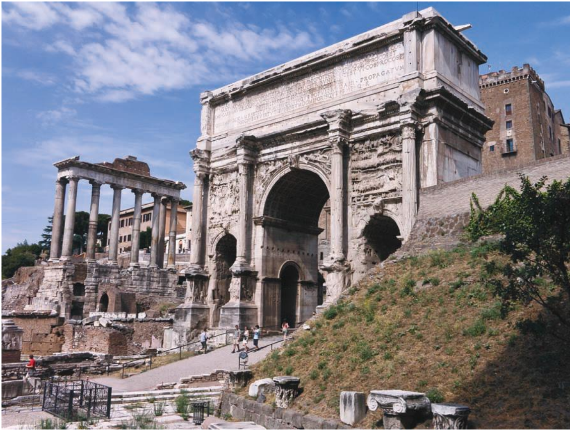
FIGURE 2.17 The 70-foot-high (21.3 m) Arch of Septimius Severus at the Forum in Rome (AD 203) is a typical Roman monument that bears inscriptions telling of an emperor's conquest. These triumphal arches were constructed of brick, travertine, and marble throughout the Roman Empire.
