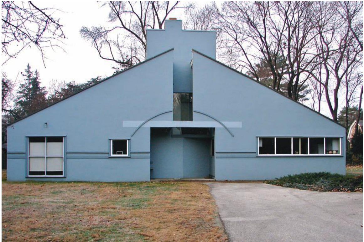
FIGURE 3.36 Venturi designed the Vanna Venturi House (1962) in Philadelphia for his mother. He manipulated various classical architectural elements such as a broken pediment entry.
