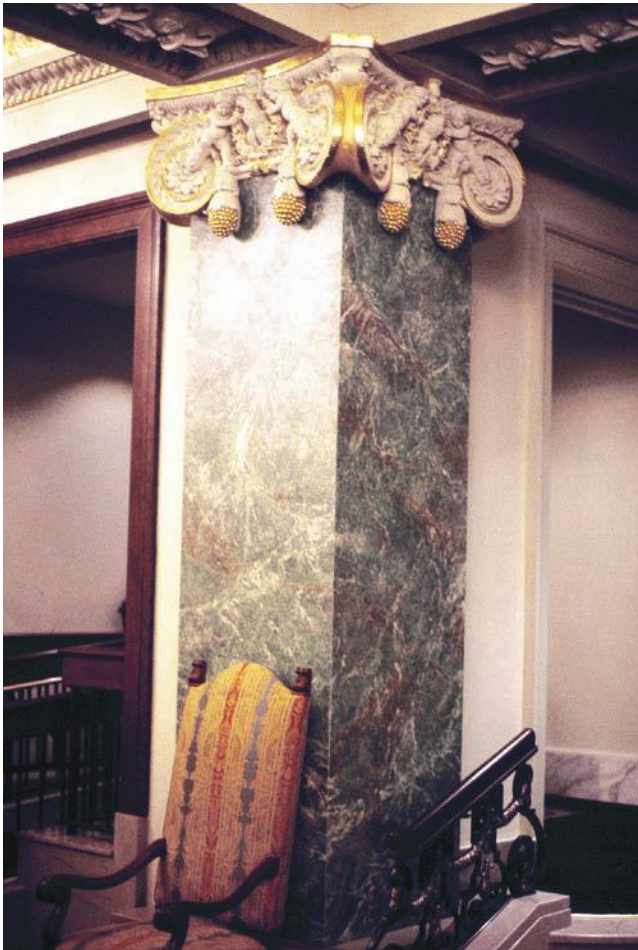
FIGURE 4.39 The patterns and texture on this column are “faux marble” as created with paint by Brett Moore of Restoration Paintwerks.
