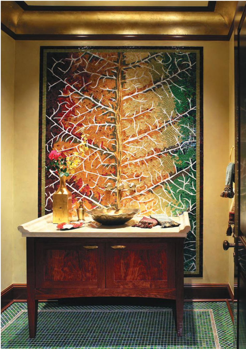
FIGURE 14.30 Small squares of tile can be used to create complex, colorful images such as this wall in a bathroom.
