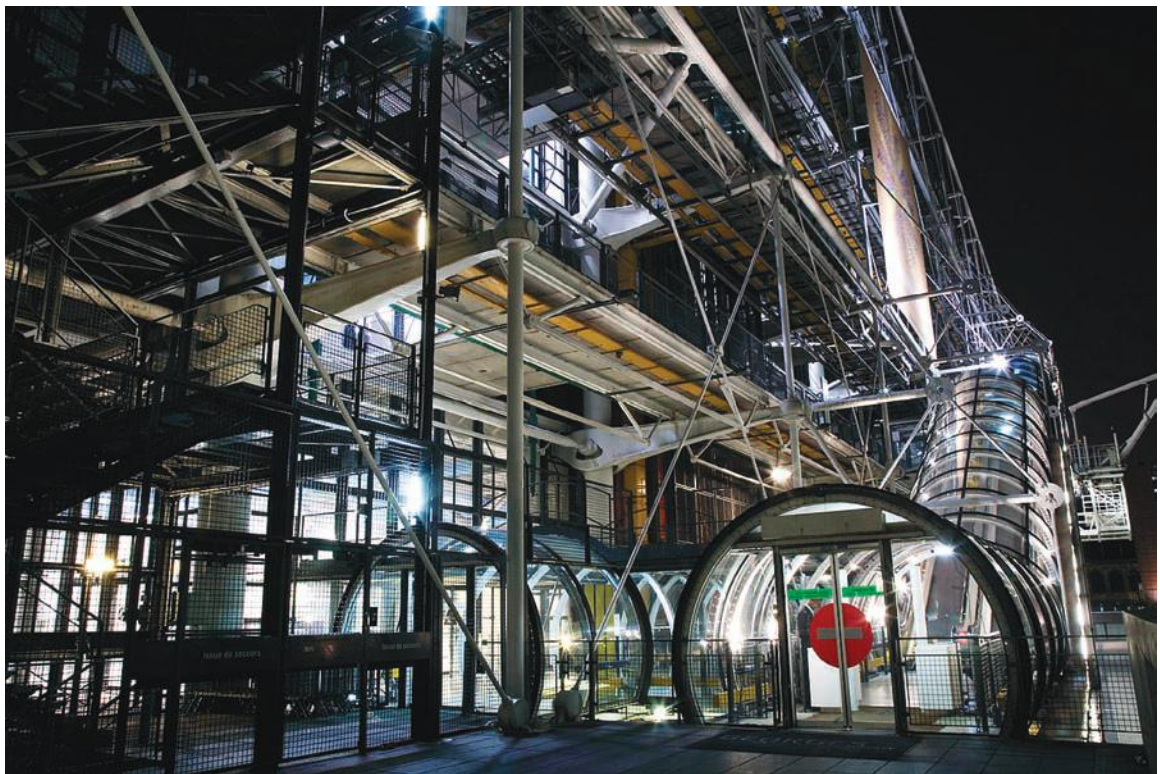
FIGURE 3.43 The Pompidou Centre in Paris is a prime example of high-tech style. It exposed and color-coded many of the building systems such as structure, mechanical, and escalators rather than hide them behind facades. CC-BY-SA-3.0/ © Jorge Royan
