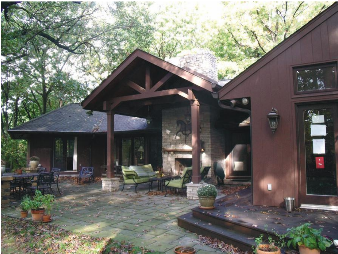
FIGURE 13.16 Sandstone is used for this outdoor fireplace addition, providing a rich textural quality to the setting.
