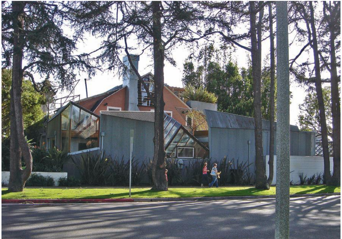
FIGURE 3.45 For his own home design in Santa Monica, California (1978), Frank Gehry clustered his architectural composition around corrugated metal, wood, and chain-link fencing. CC-BY-SA-2.0/IK's World Trip
