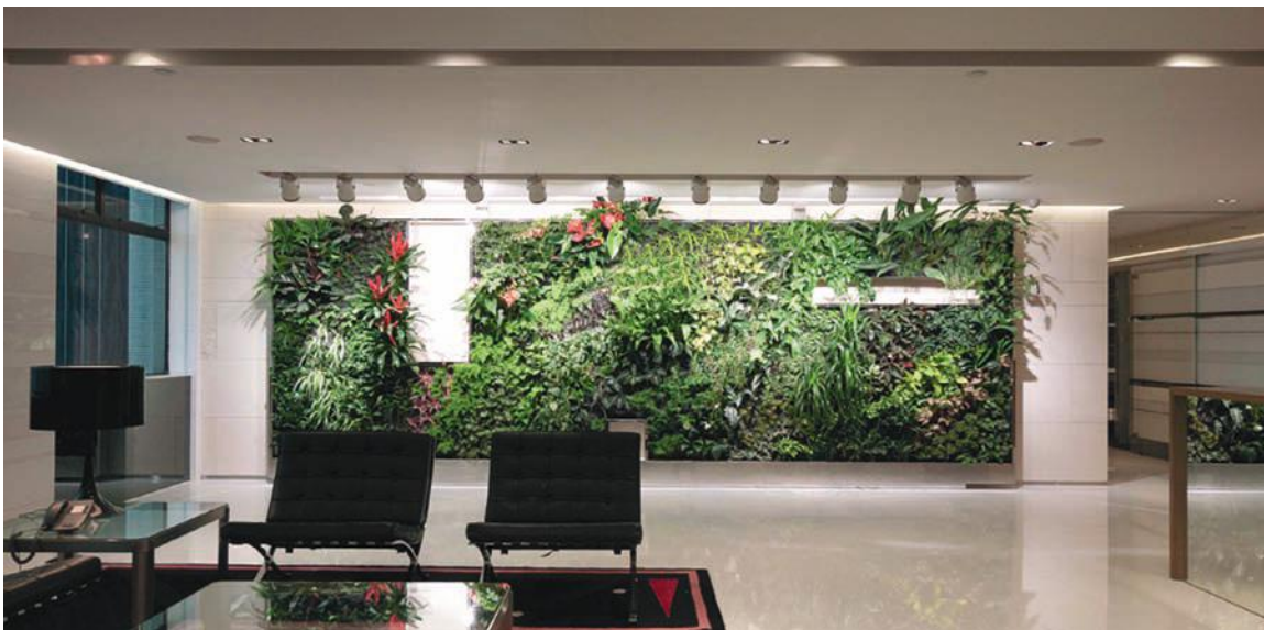
FIGURE 3.56 This biowall uses plants to clean the indoor air through a filtering process. It also adds closeness to nature, by introducing it into the architecture of the building.
