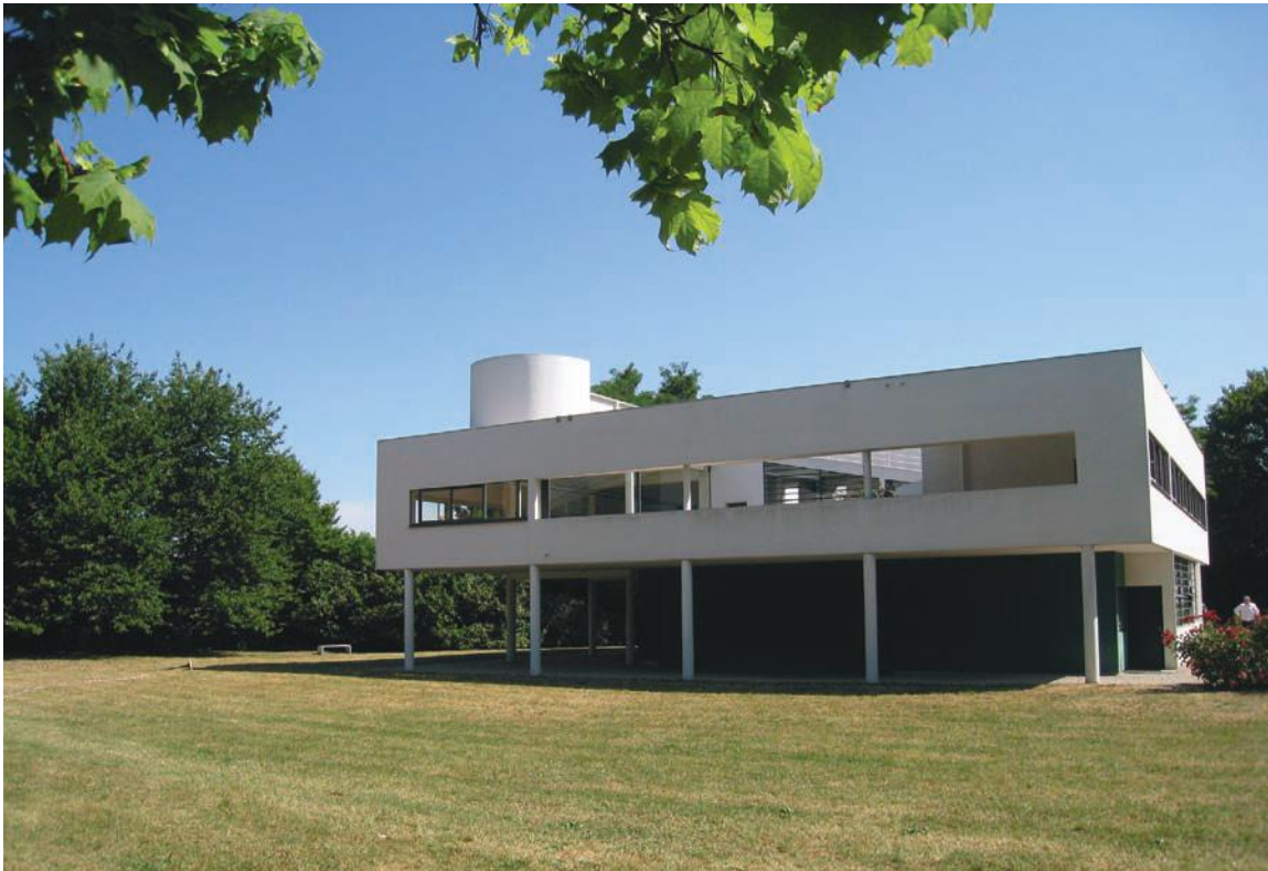
FIGURE 3.14 Le Corbusier, with Pierre Jeanneret, designed the Villa Savoye (1929–1930) in Poissy, France (near Paris), in the simple, geometric forms of the Modern style. The main living area of the house is raised above the ground-level garage and entry foyer. The roof is provided with a patio and protected by a windscreen.
