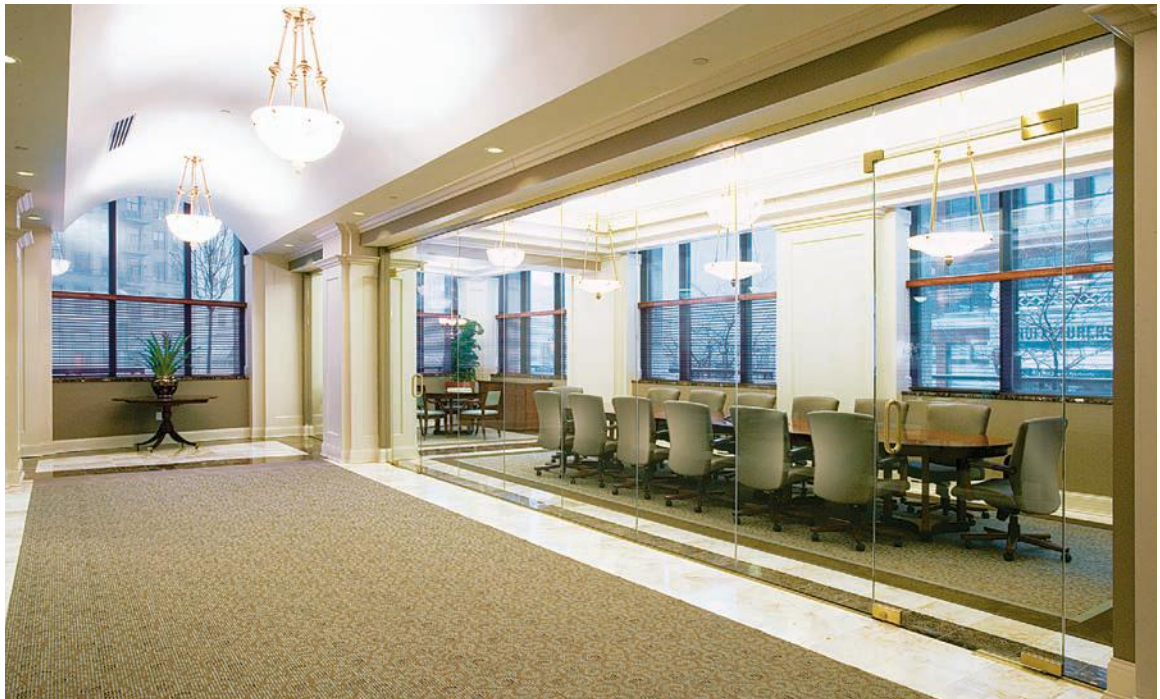
FIGURE 15.7 Large glass doors at the ends of this conference room glass wall match the frameless glass sections. Courtesy of Kimball Office.
