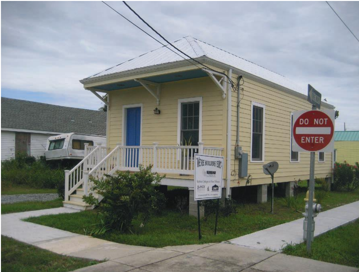
FIGURE 3.58 The Katrina Cottages are small residential structures that are now designed and marketed across the United States, as interest in small dwellings becomes more prevalent.
