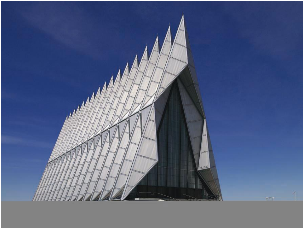
FIGURE 4.34 The triangular shapes in the Air Force Academy Chapel, Colorado Springs, Colorado, exhibit very dynamic shapes and contrasting angles. It emphasizes stability by its broad base as its apexes point upward.
