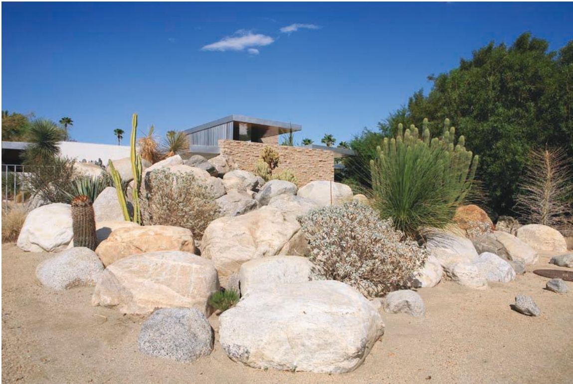
FIGURE 3.29 The Kaufman House (1946) in Palm Springs, California, was designed by Richard Neutra. It is a prime example of modernism.
