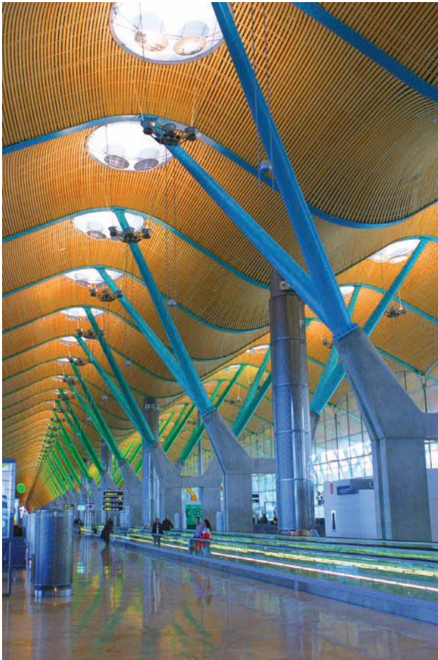
FIGURE 4.49 The large tree-like columns and the curved beams they support in the terminal at Barajas Airport (Madrid, Spain) provide an emphasis in color and form to the space.
