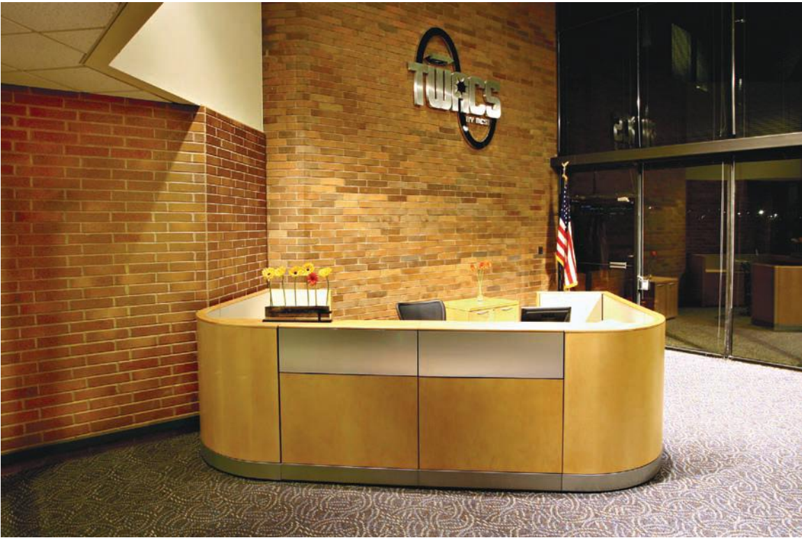
FIGURE 13.21 These two brick walls in this reception area are laid with different brick types, bonding methods, and surface finishes. Courtesy of Kimball Office.
