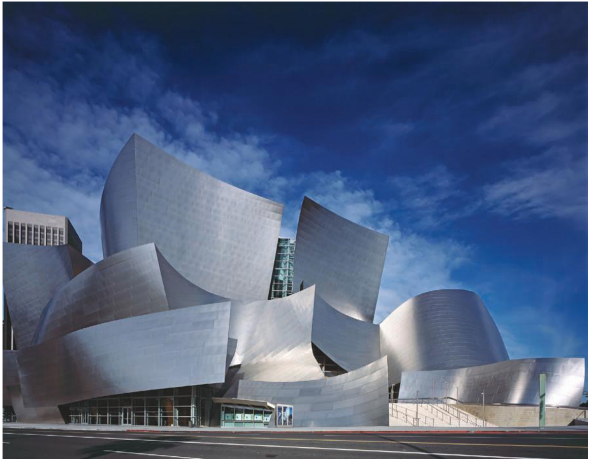
FIGURE 3.54 Frank O. Gehry designed the Walt Disney Concert Hall for the home of the Los Angeles Philharmonic utilizing CATIA (computer-aided three-dimensional interactive application) for the complex shapes and construction.
