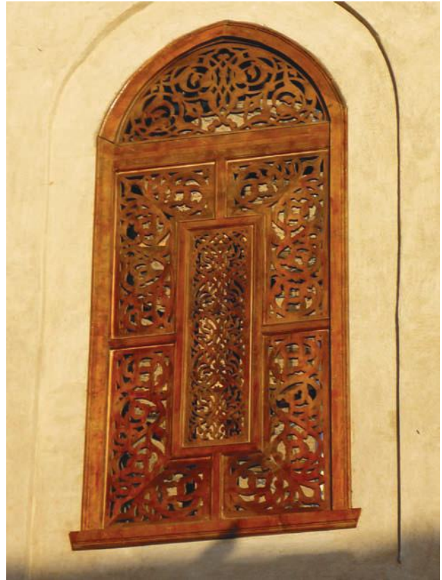
FIGURE 2.62 A carved wooden window grille, called a mashrabiya , can sometimes be found on a projecting second-floor window.
