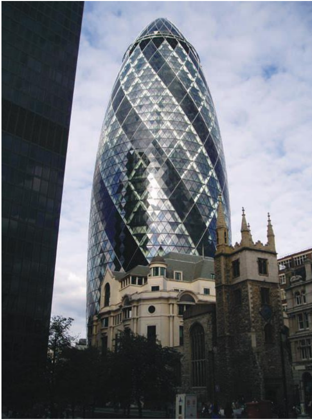
FIGURE 3.55 The building 30 St Mary Axe, London (2003), was designed to use half the power of a similar skyscraper, utilizing natural ventilation and other energy-saving techniques. Courtesy of Steve Cadman
