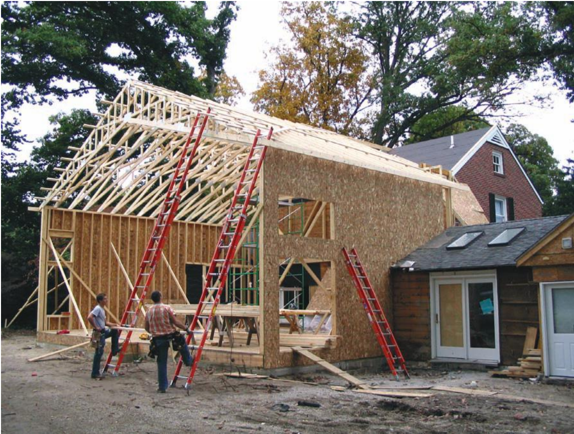
FIGURE 13.9 Oriented strand board (OSB) is used for the wall and roof sheathing of this residential addition.
