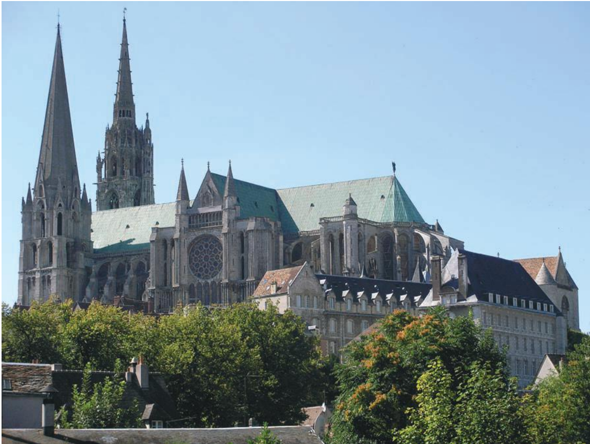
FIGURE 2.8 Chartres Cathedral (c. 1194) exhibits many features typical of the Gothic style of architecture. Pointed arches, flying buttresses, and vertical expression of structure are all characteristic of this style.
