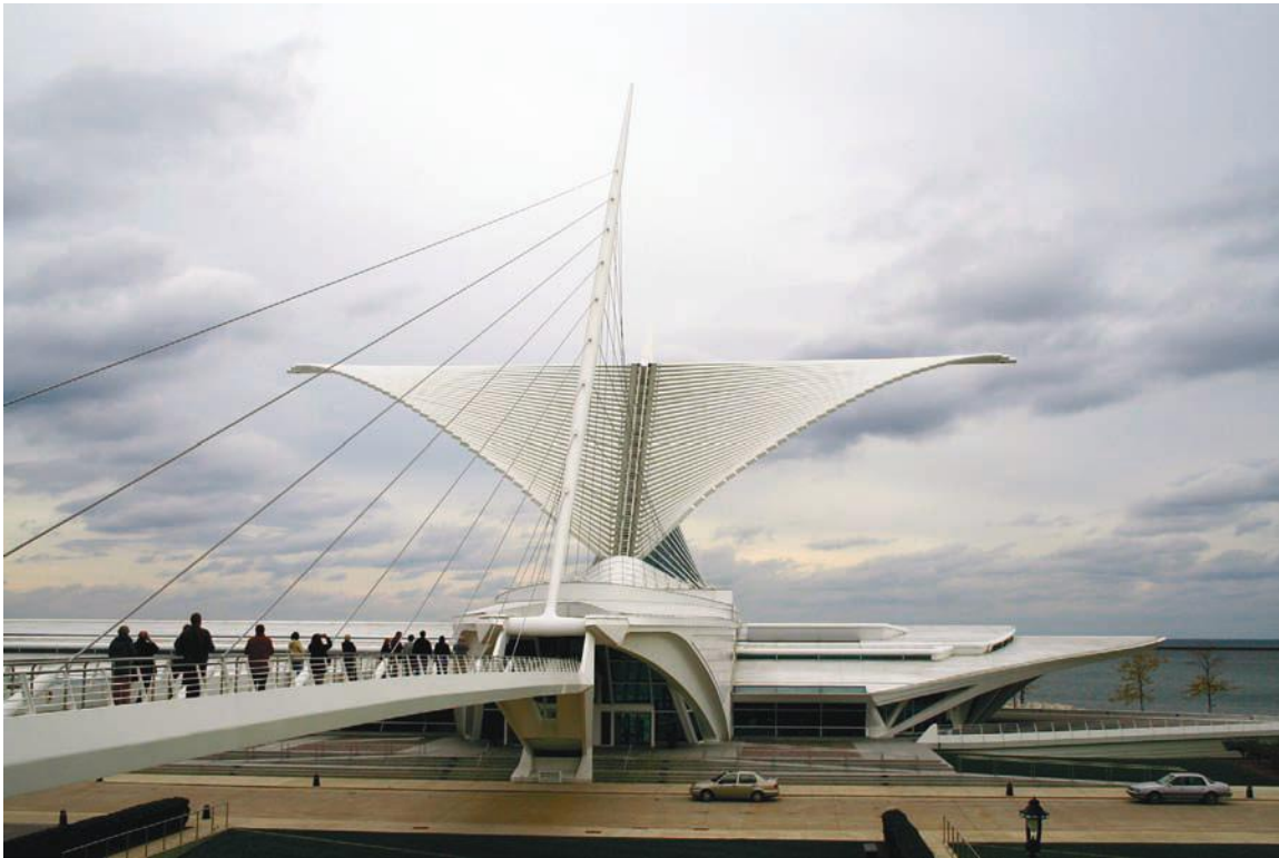
FIGURE 3.47 Santiago Calatrava designed the Reiman Pedestrian Bridge (a cable-stayed structure) in 2001, connecting the Milwaukee Art Museum on the lakeshore to the downtown’s central business district Milwaukee Art Museum.
