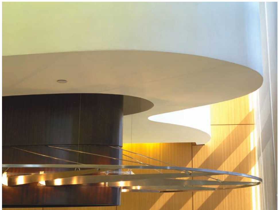
FIGURE 13.29 Stainless steel is used in custom-made curvilinear shapes in this hanging light fixture, complementing the shapes of the curved ceiling soffits.
