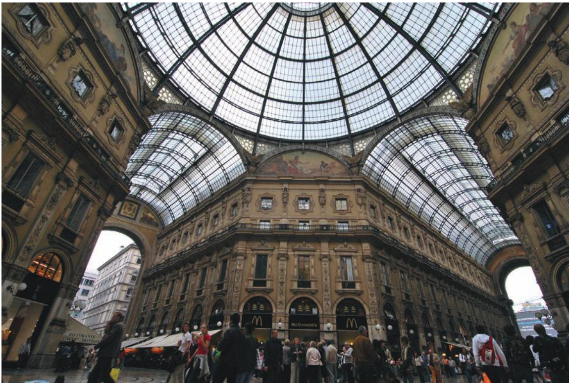
FIGURE 4.19 The two intersecting barrel vaults over the streets in the Galleria Vittorio Emanuele II, in Milan, are interconnected with a glass dome, creating a distinct spatial feature.
