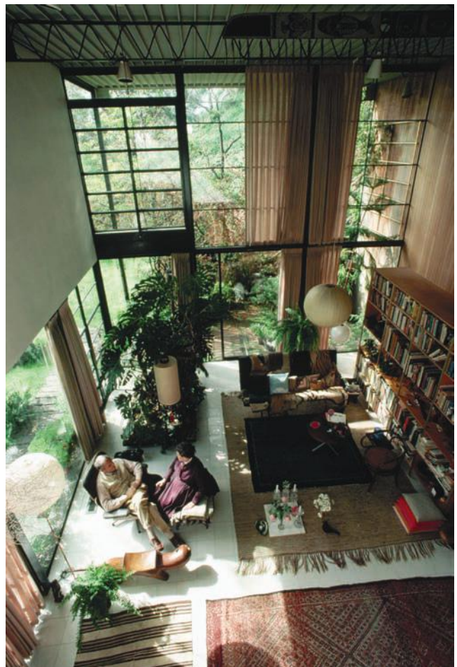
FIGURE 3.25 Charles Eames built his own home (1949) near Los Angeles of modular lightweight steel framing members. These systems allowed a great flexibility in placement of windows, walls, and other components.
