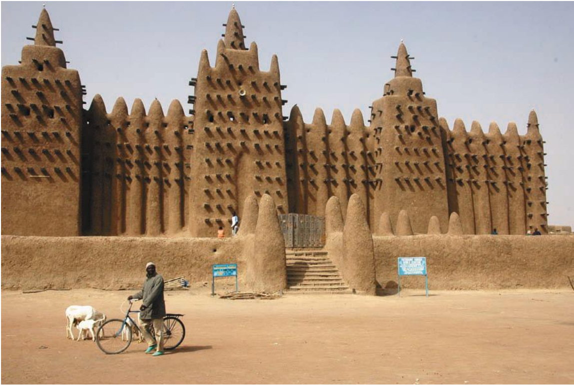
FIGURE 2.56 The mud mosque of Djenné is the largest mud brick building in the world and one of the most famous landmarks in Africa.
