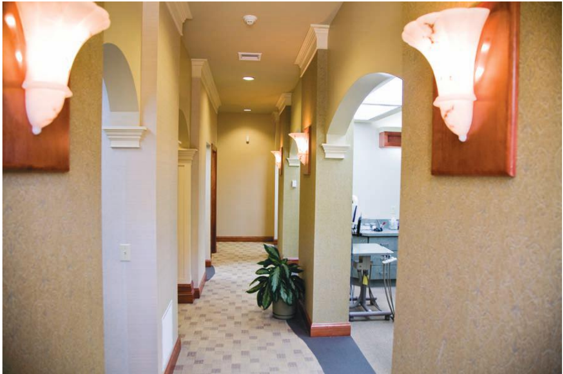
FIGURE 12.38 The use of wall sconces in the corridor of this dental office provides general lighting and serves as accent lighting.
