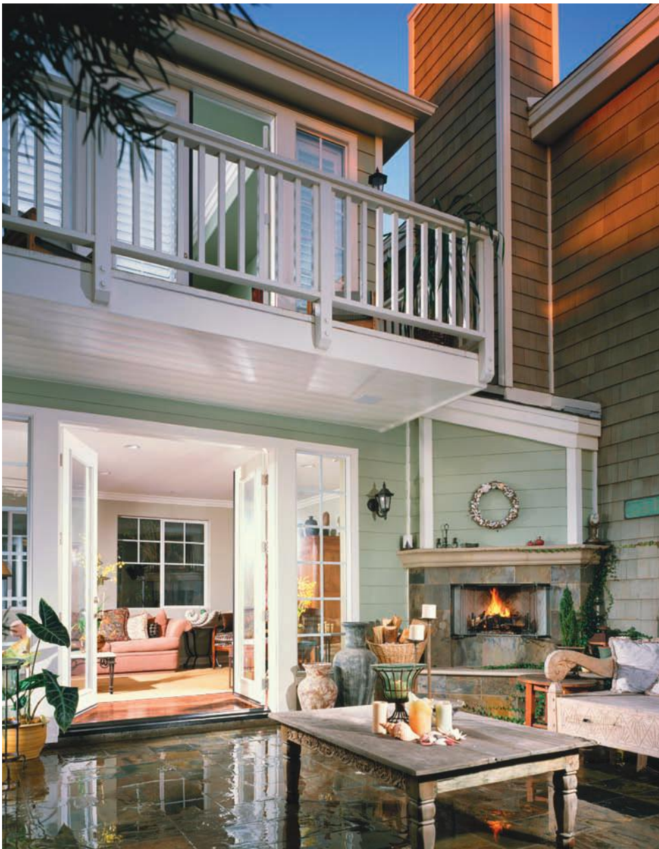
FIGURE 13.3 Wood has good properties to be used in framing the cantilever construction in this balcony.
