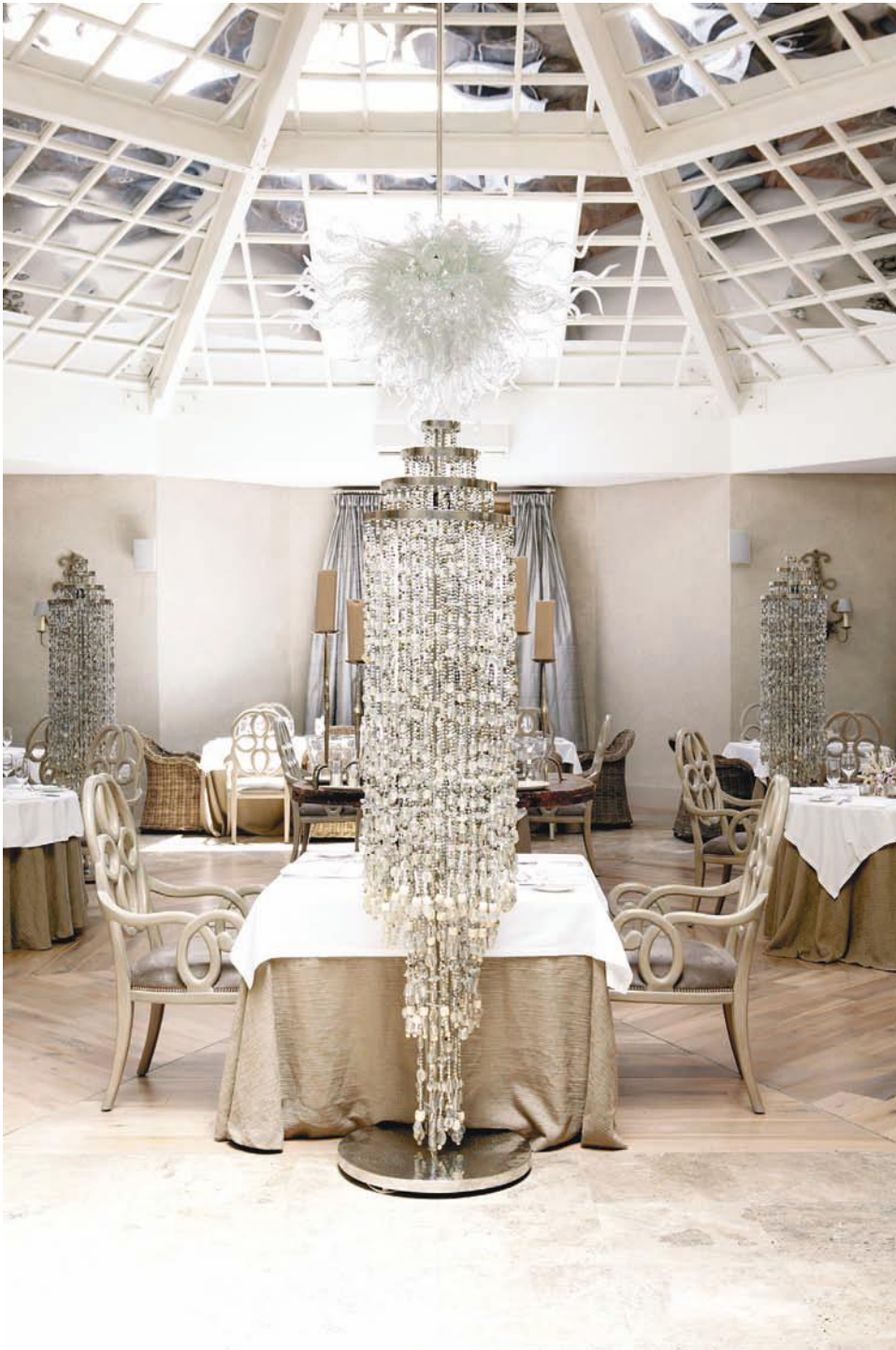
FIGURE 14.34 The ceiling in this restaurant is constructed of varying grid shapes and mirrors to reflect light and images throughout the space.
