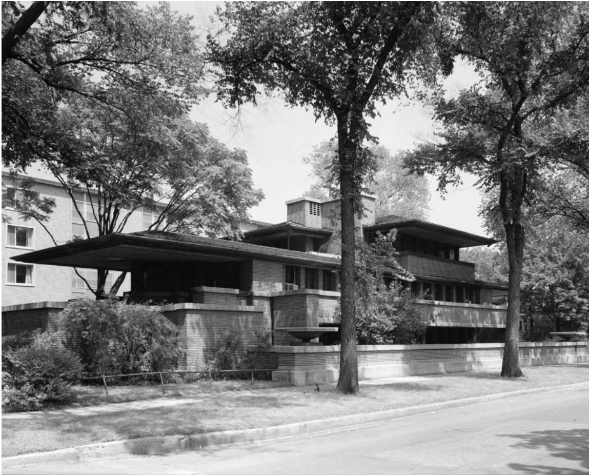
FIGURE 3.11 Frank Lloyd Wright’s design for the Robie house (1909) in Chicago exhibits long horizontal flowing forms extended from a central fireplace core.
