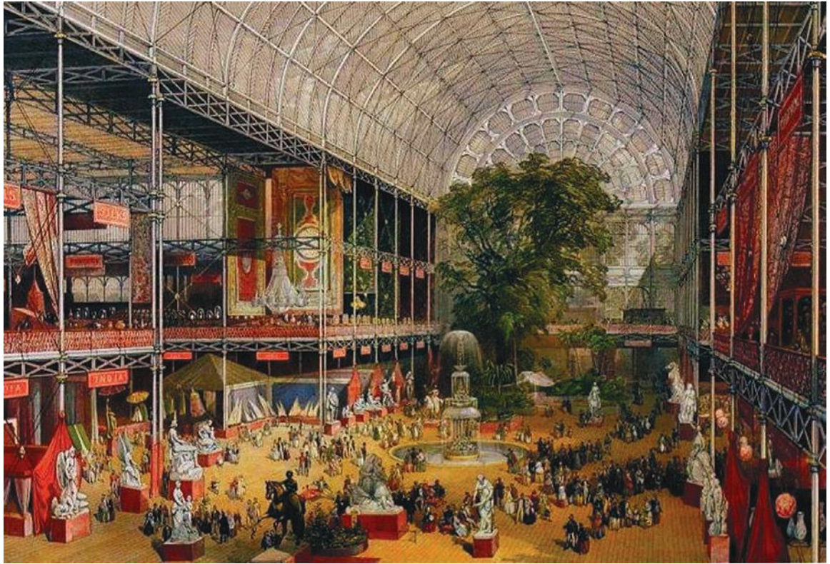
FIGURE 2.55 The Crystal Palace, designed by Joseph Paxton, was a prefabricated iron-and-glass structure that housed the first World Fair, the Great Exhibition of 1851. It was over 1,848 feet (564 meters) long, and 454 feet (138 meters) wide.
