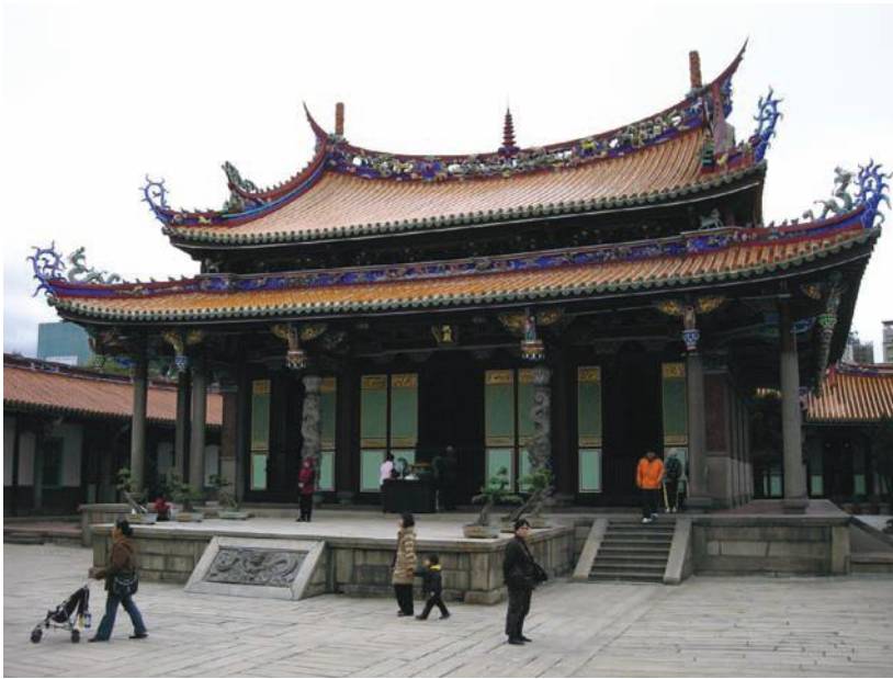
FIGURE 2.63 The Chinese timber technology can be seen in the Teipei Confucius Temple located in Taiwan. The temple was built in 1854, destroyed in 1895, and rebuilt in 1925.
