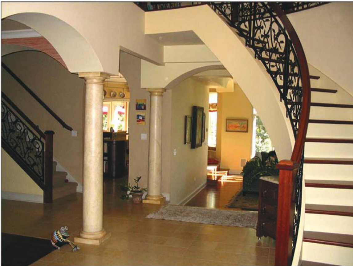
FIGURE 2.14 The columns in this new residence are inspired by classical Doric orders of Greek and Roman architecture.
