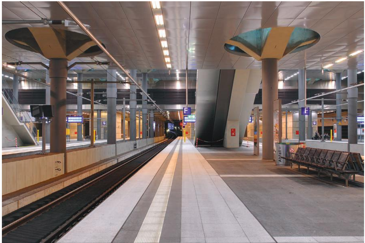
FIGURE 4.30 The Berlin Central Railway Station is designed with strong geometrically derived structural shapes and finishes. CC-BY-SA-3.0/Mihael Grmek
