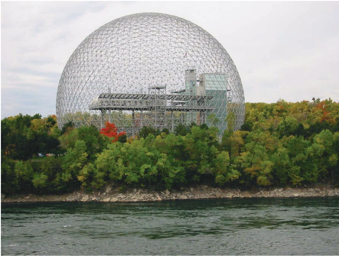
FIGURE 4.2 The framework of Buckminster Fuller's geodesic domes is established by mathematical proportions and structural analysis. This is a good example of the structural design approach.
