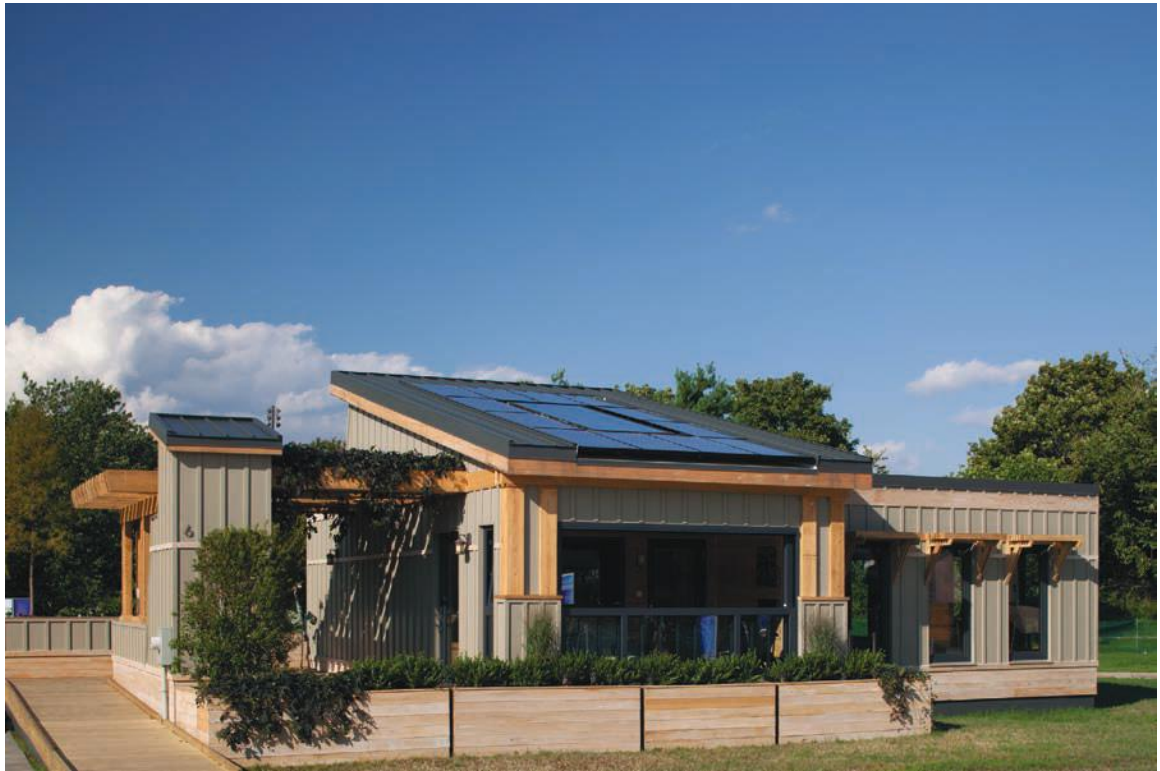
FIGURE 11.12 These photovoltaic panels supply more electricity to this small house than it needs, resulting in a “net zero energy usage.”
