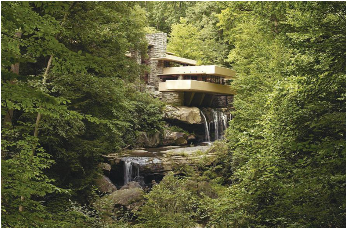
FIGURE 3.13 Wright designed Fallingwater to sit over a stream and waterfall. It is composed of a series of cantilevered terraces and balconies with concrete as the horizontal elements and limestone for the vertical ones.
