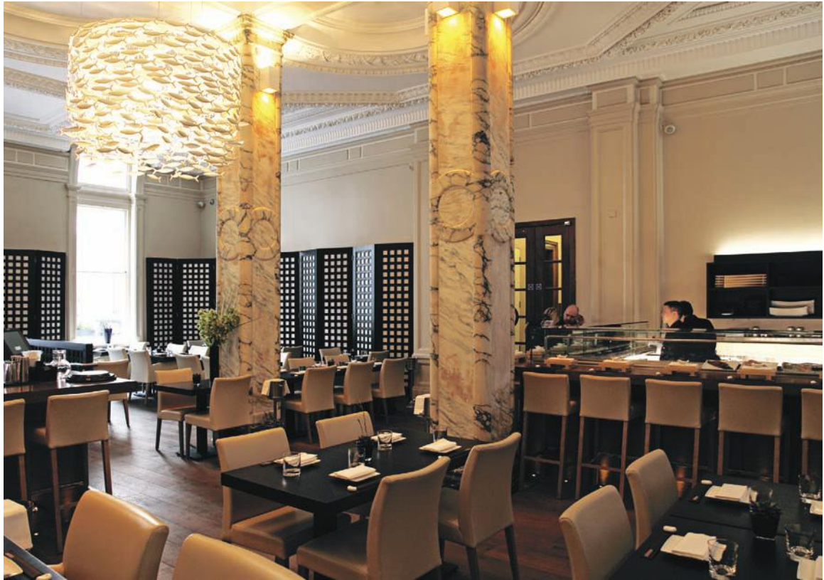
FIGURE 13.23 The ornate ceiling and pilasters in this restaurant are created with plaster work.
