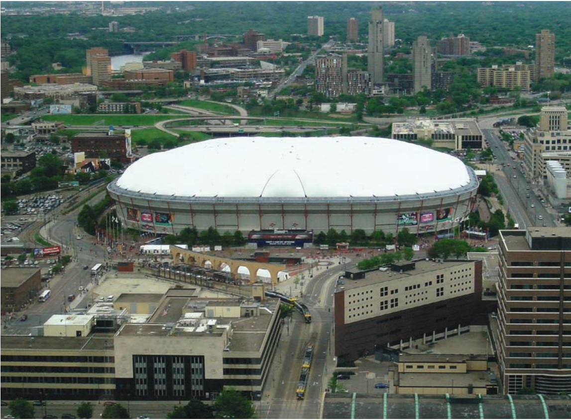
FIGURE 14.10 The Hubert H. Humphrey Metrodome is a tensile structure constructed of fabric reinforced with steel cables and inflated with air.
