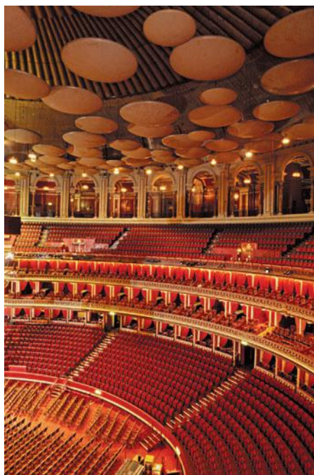
FIGURE 11.24 The interior of the Royal Albert Hall in London features large saucers that are installed near the ceiling to improve acoustics of performances and to combat echo problems. Lebrecht Music and Arts Photo Library/Alamy
