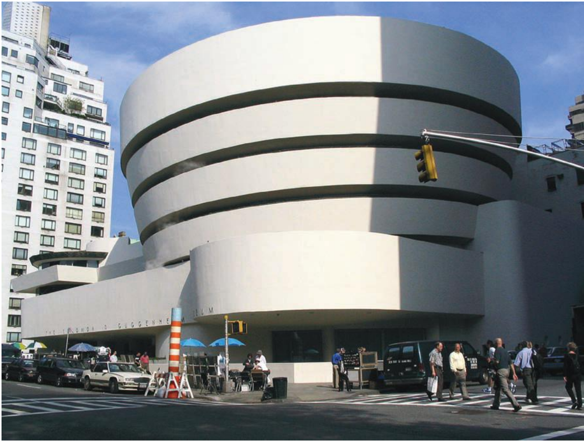
FIGURE 3.35 The Solomon R. Guggenheim Museum (1956–1959) in New York by Frank Lloyd Wright. This fluid, reinforced concrete structure is dominated by the creation of the large central spiral ramp.
